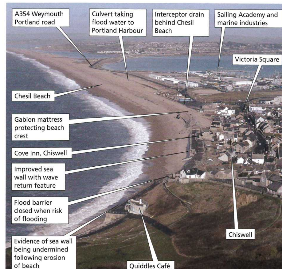
Photograph 1 Annotated photo of southern end of Chesil Beach showing the features mentioned in the text
